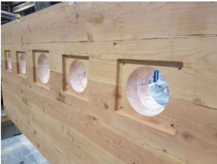
Pictured above: Stop Log Panel
