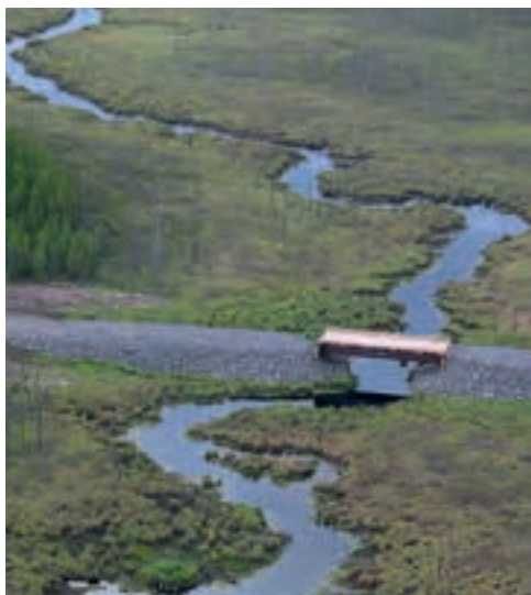
FIGURE 69. A bridge is used to cross a channel where a culvert is not well-suited.
