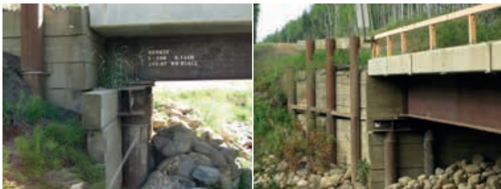
FIGURE 67. A pile-supported abutment (left) and a pile-supported wingwall (right).
