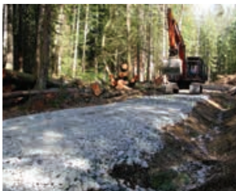
FIGURE 83. The use of an aggregate running surface protects the underlying soil from erosion.
