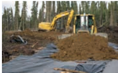
FIGURE 32. Bulldozer working on top of a positioned corduroy structure as it delivers a layer of fill.
