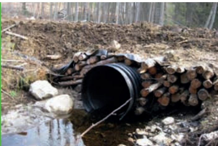
FIGURE 46. Logs placed on either side and over the top of a culvert. Notice the placement of the geotextile separation layer over the parts of the logs that are exposed, which prevents road material from eroding into the watercourse.
