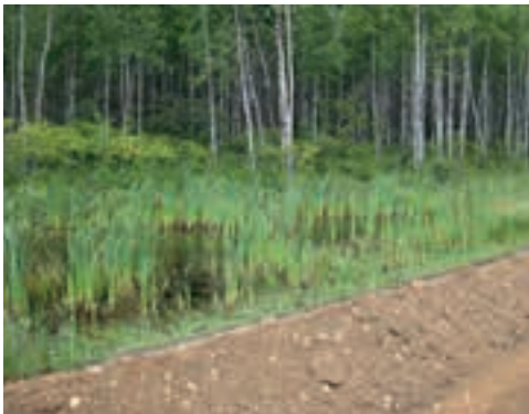
FIGURE 79. Blockage of wetland flow can result in water ponding and negative impacts to the road base.
