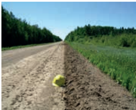
FIGURE 84. Berm of material near the shoulder of the road developed by a grader will be worked back across the road to build a crown. Careful attention must be given to the protection of roadside vegetation.
