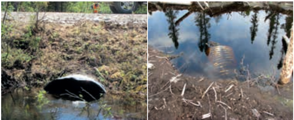
FIGURE 43. Culverts that have sunk below the water surface.
