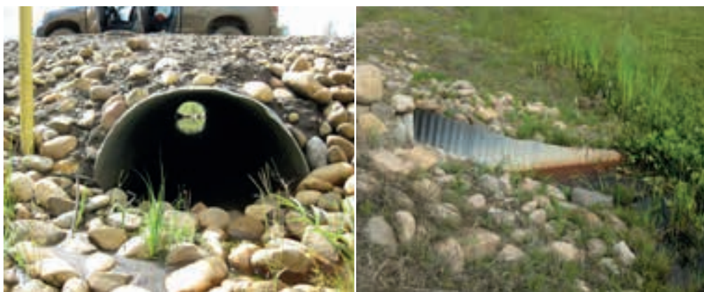
FIGURE 42. A partially embedded culvert (left) and a culvert prepared with a step-bevel (right).
