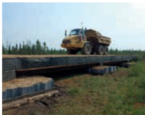
FIGURE 61. A pile-supported jump span bridge allows the road to span open water and sensitive wetland sites. (Photo courtesy of Landmark Solutions.)
