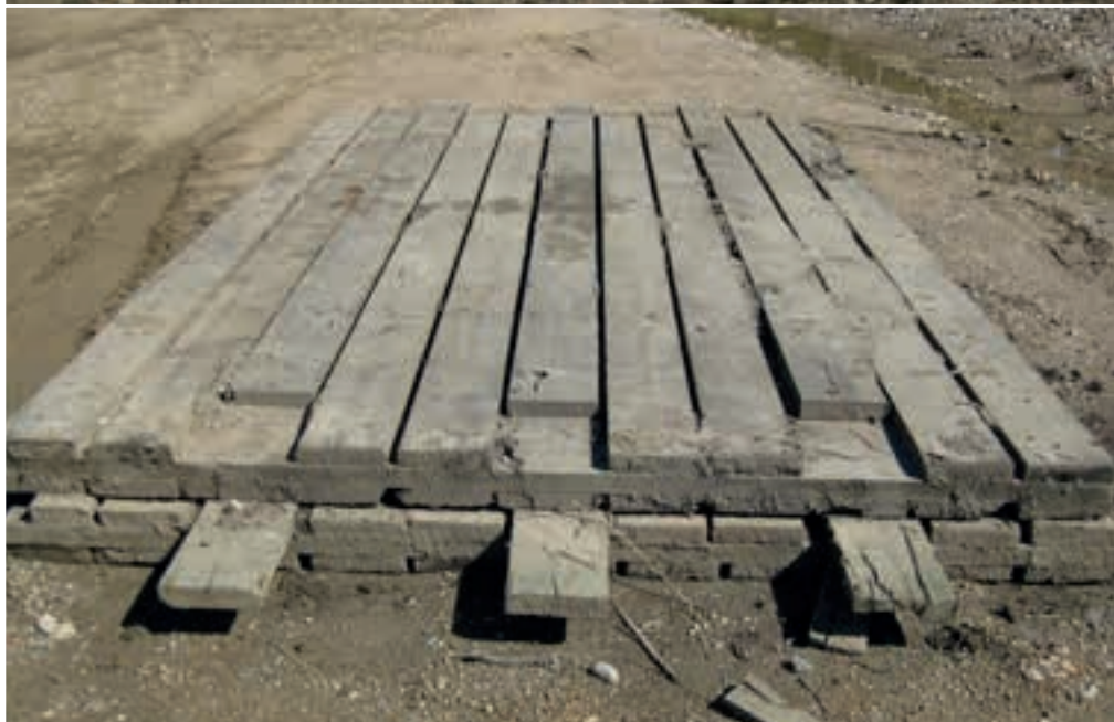
FIGURE 39. Temporary mats made of wood and metal (top) and all wood (bottom). Note that the two all-wood mats stored on top of each other have a three-finger interlock design for joining with adjacent mats when positioned end-to-end.
