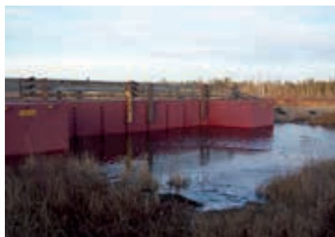
FIGURE 68. A floating bridge alleviates some of the load-bearing requirements associated with typical abutments. Here, a floating bridge was chosen to cross a defined channel through a wetland as the channel did not freeze to the bottom during winter access, and seasonal timing was not always conducive to the construction of an ice bridge.
