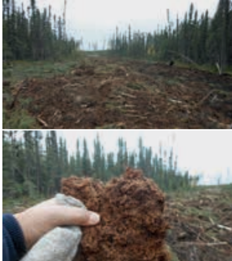
FIGURE 23. A recently cleared wetland crossing showing minimal disturbance to the root mat and peat layers (top) and a close-up of typical peat (bottom).
