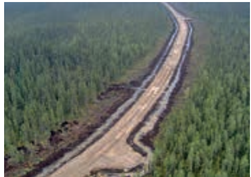
FIGURE 80. Permanently filled ditches can be a consequence in certain wetland types and can negatively impact road performance. (Photo courtesy of Tembec.)
