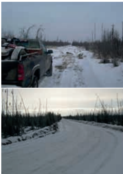
FIGURE 41. Winter roads across frozen wetlands can have a much lighter impact on the surface vegetation and soil if constructed and used appropriately, resulting in less rutting and compaction.
