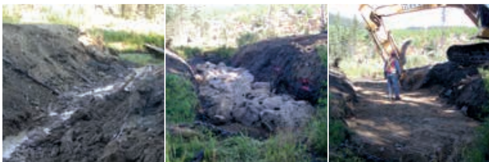
FIGURE 66. A sequence of events for improving the bearing capacity of a site in preparation for installing an open-bottom arch. The weak soil was identified as not meeting the design requirements for corrugated pad footings (left); large aggregate was placed after excavation of weak soil (middle); coarse sand was used to level the site in preparation for the placement of the open-bottom arch (right). The stream was then diverted back through the arch.
