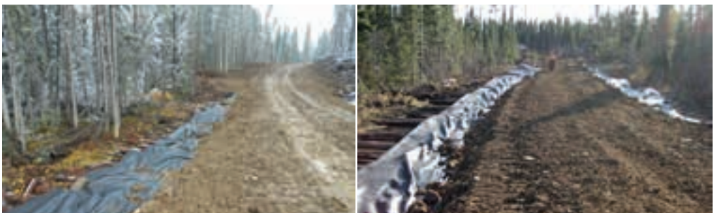
FIGURE 56. Two corduroy roads showing the use of logs, a separation layer, and road fill as part of a road across a wetland.
