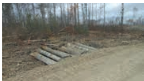
FIGURE 51. Log bundle installed through a temporary road across a shrub swamp. The structure is built one log high, with a separation layer above the logs and the road material. Note that culverts are easily incorporated into this style of structure.
