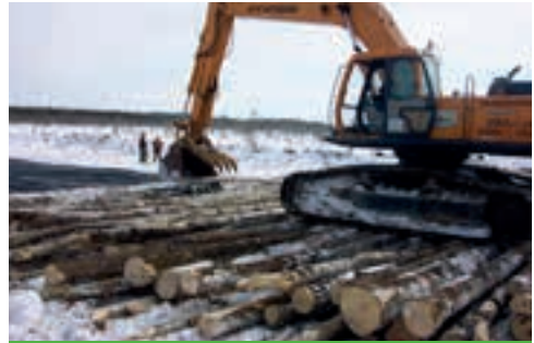
FIGURE 33. A section of corduroy being built with larger-diameter, tree-length logs more than one log high. Notice the alternating directions of butts and tops to make the structure level, as well as the use of geotextile below the logs.
