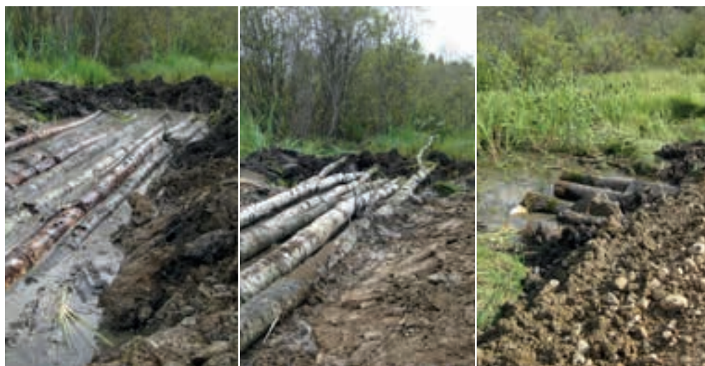
FIGURE 52. First row of a log bundle in an excavated trench (left); second row of the log bundle before the tops of the logs were trimmed (middle); final road grade showing the log bundle with geotextile placed over it (right). Note that this log bundle was installed through an existing road to provide additional water passage.
