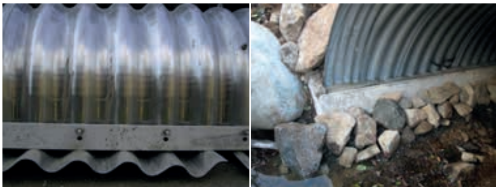
FIGURE 65. Typical footings for an open-bottom arch: a corrugated pad footing (left) and a precast concrete footing (right).
