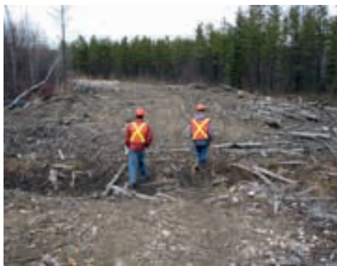
FIGURE 82. The removal of conduits and trenching across the road can aid in restoring natural surface and subsurface wetland flow.
