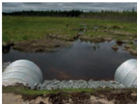
FIGURE 45. Closely spaced culverts that balance flow on either side of the road at a wetland location where sections of open water are present. (Photo courtesy of Tembec.)
