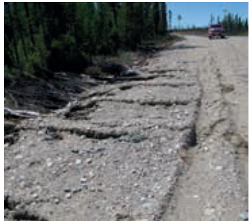
FIGURE 77. Uneven road surfaces can be an indicator of road settlement.
