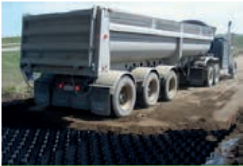
FIGURE 30. Perforated geocells stabilize and confine fill material. They are often applied when high loading is expected and where granular material is unavailable. (Photo courtesy of Presto Geosystems.)
