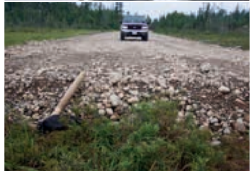
FIGURE 34. Construction of a corduroy section of road during the winter, with geotextile being placed along the ground surface (top). The completed road crossing, which was built with delivered aggregate (bottom).
