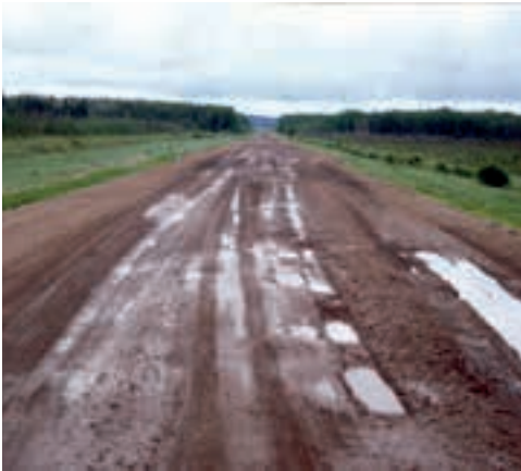
FIGURE 74. Rutting of the road surface can be an indicator of problems with the underlying road layers.
