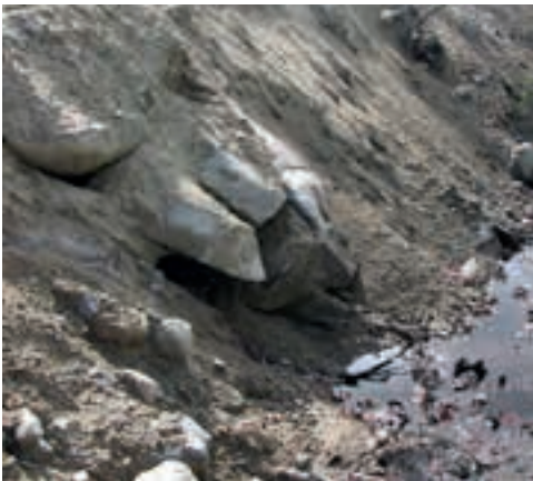
FIGURE 76. Erosion from road embankments can block culverts and impede water movement.
