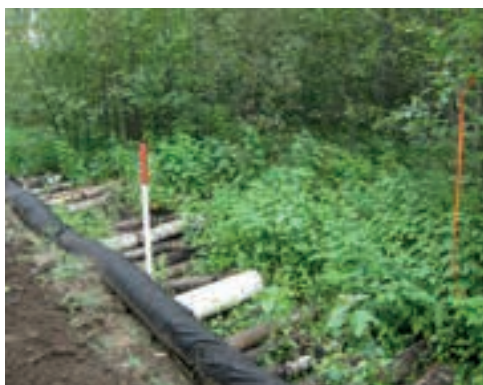
FIGURE 60. A culvert was incorporated into this corduroy crossing to provide for additional flow capacity. The culvert was positioned at a low area, where greater flow was anticipated. Note that the geotextile used for separation has been secured by wrapping it around a curb log.
