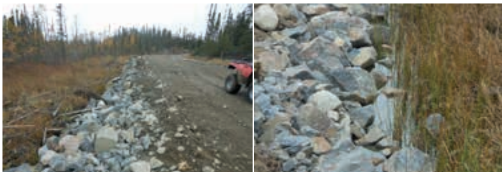
FIGURE 54. Newly built resource road across a wetland showing the size and depth of rocks used for the aggregate mattress.
