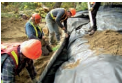
FIGURE 81. A woven geotextile is attached to dimensioned lumber to aid in removal during road decommissioning.
